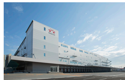
Automation enables the Saitama ALC to provide rapid, superior one-stop logistics services for a lineup of over 30,000 products
