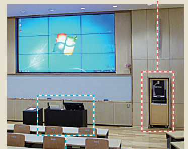
The video source devices, such as the BD player and document camera, are mounted in the rack together with other video devices. The rack is recessed in the front wall of each lecture hall, and the door can be opened for access whenever necessary. The rack can be pulled out from the wall for maintenance.
