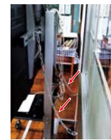
◀ In order to prevent the electronic blackboard from falling over in the event of an earthquake, it is fixed to the wall with chains (red arrows) when not in use.
