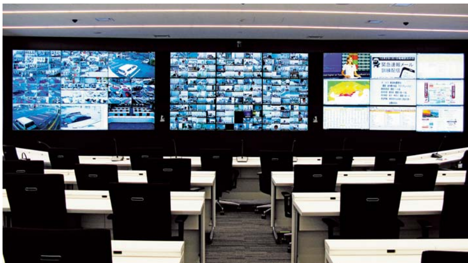
The multiscreen system, made up of 27 55-inch LCD displays, lets you view a wide range of information with one glance.
