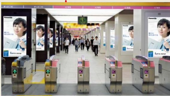
▲ In the passageway to the ticket gates, 70-inch high-definition LCD displays are installed, utilizing the entire column width. A series of 20 displays, each showing crisp, high-luminosity images, draws station users' attention and delivers ad messages effectively.
