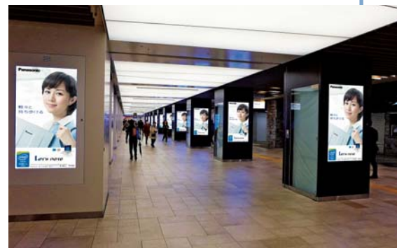
70-inch full high-definition LCD displays are mounted on the columns in the passageway leading to the ticket gates, which are slightly thinner. Because the flow of pedestrian traffic moves in a straight line, displays are mounted on two sides of the columns.
