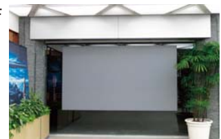
The projector and transmissive glass-window screen installed in the 1st floor lobby.
