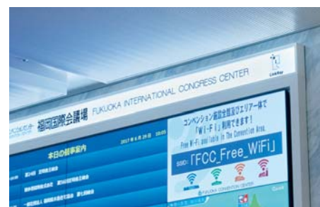
The top part of the display panel is installed with a LinkRay Light ID transmitter. Use of this device in the future is expected to deliver information with even higher added value.
