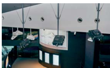
▲ The closely suspended projectors at the exhibition zone. By using both white and black cabinets according to the color of the ceiling materials, they appear harmonious with the surrounding architecture. The wall surfaces and ceiling are also inclined, so there are no projectors that are suspended at the same angle or height. During the construction of the site, 3D simulations were carefully conducted.
