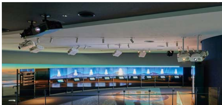
▲ The closely suspended projectors at the exhibition zone. By using both white and black cabinets according to the color of the ceiling materials, they appear harmonious with the surrounding architecture. The wall surfaces and ceiling are also inclined, so there are no projectors that are suspended at the same angle or height. During the construction of the site, 3D simulations were carefully conducted.
