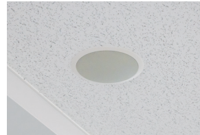
▲ RAMSA Near Field Speakers are installed as auxiliary speakers to cover the central area of the classroom. (Ceiling Embedded) WS-AC066
