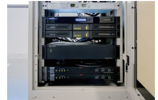
▲ The acoustic rack contains two RAMSA Digital Power Amp WP-DM912 units, which can automatically run the calculated values processed by PASD.
