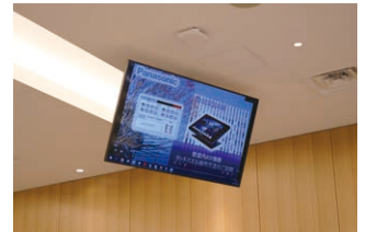
▲ Eight TH-65EQ1 65-inch 4K UHD LCD Displays are installed in the large lecture hall
