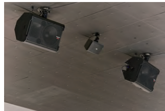
▲2-way speakers were applied inside the pavilion to realize powerful sound staging
