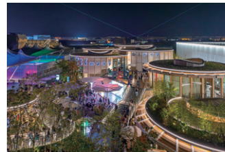
▲ Night view of the pavilion, constructed from wooden prefabricated structures and rented steel, including materials used here for the first time.
