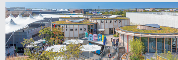
▲ The pavilion is composed of two buildings—the themed exhibition area and the restaurant—forming an ensemble. Seven circular timber structures are arranged with cylindrical units connected to each circle.
